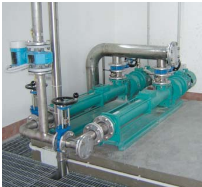
Vaste water plant: pumps in operation to feed a centrifuge-decanter
